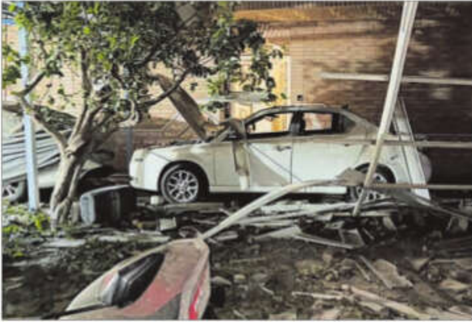
Debris surrounds a car at the site of US strike in Kuhestak, southern Iran, on Wednesday. REUTERS
